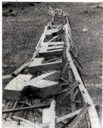
TOWER of KELK Elko, Nev., looked like this after an 80-mile-an-hour gale hit it last month. Van Welch, station's chief engineer, reports KELK was back on air with temporary antenna less than 10 hours after tower went down. KELK is erecting new 200-ft. permanent tower. Station operates with 250 w unlimited on 1340 kc.
